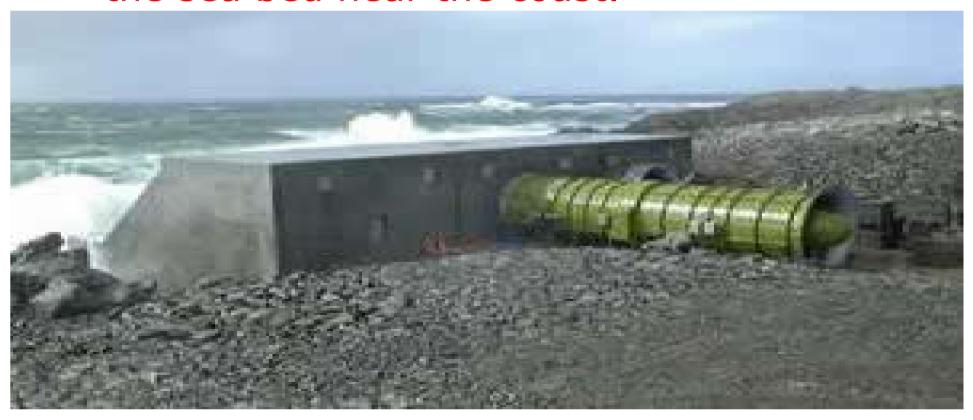
Waves passing across the top of the unit make a piston move, which pumps seawater to drive generators on land. They're also involved with wind power and biofuel.
